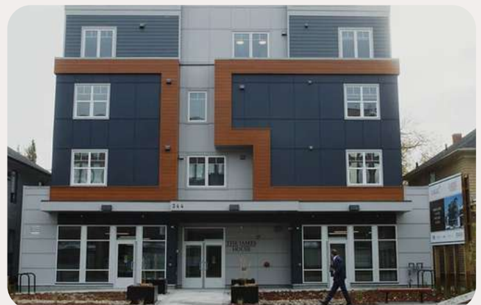
The James House. Source: McMan Calgary (2020).
